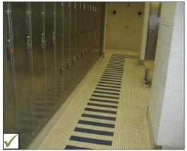
Consistent accessible path of travel, space for circulation and lockers mounted at different heights.
