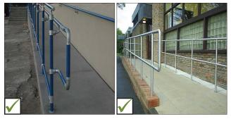
Ensure handrail extensions do not obstruct path of travel or create hazards.
