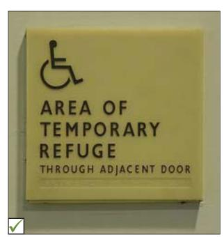
'Areas of Refuge' should be designated with signage, including Braille and tactile features for users with vision loss.
