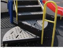
Transfer system to connect elevated play components.
