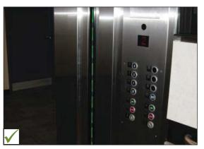
Elevator sensor door and floor registration buttons.
